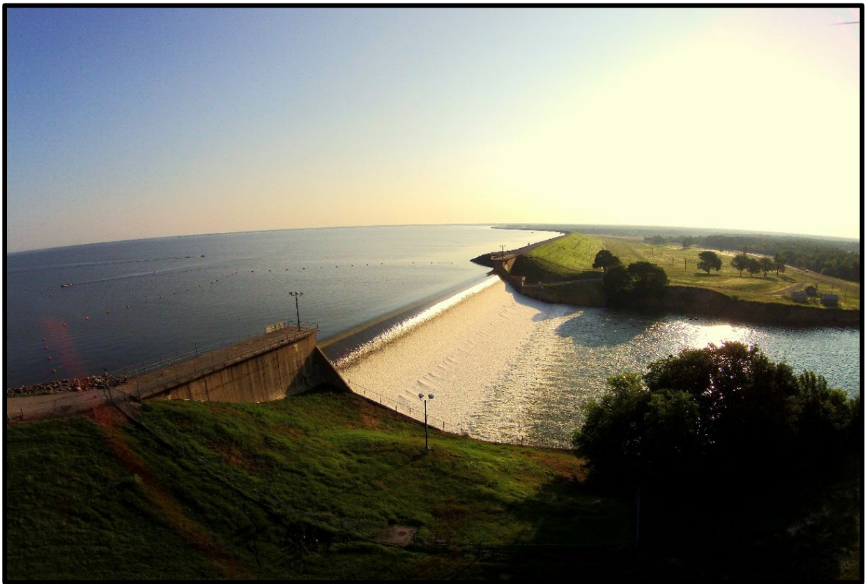
Figure 2. Lake Tawakoni ungated concrete spillway.
