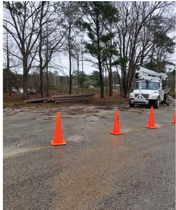
Figure 2: Undeveloped area being cleared.
