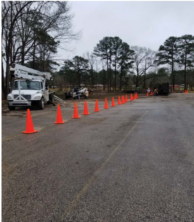
Figure 1: Current paved area
