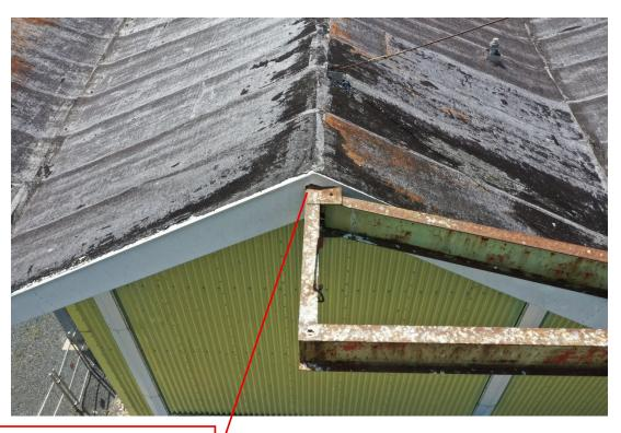
Remove existing Steel Beams, at roof clip. Roof clip to remain. Contractor to prepare surface and apply Amide Epoxy Paint System (typical all locations).
