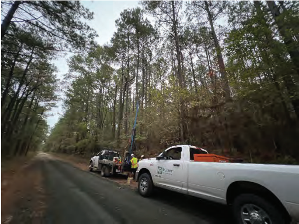
Facing Northeast at Boring B-01
