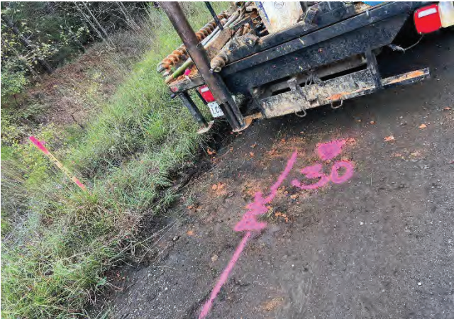
Facing Southeast at Boring B-30
