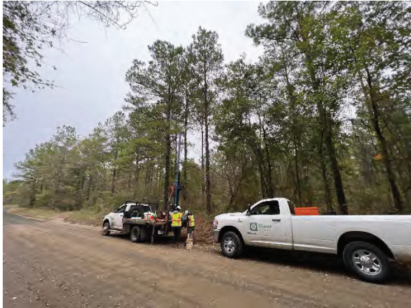
Facing Northeast at Boring B-03
