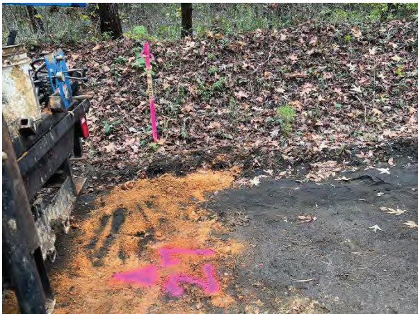
Facing East at Boring B-27
