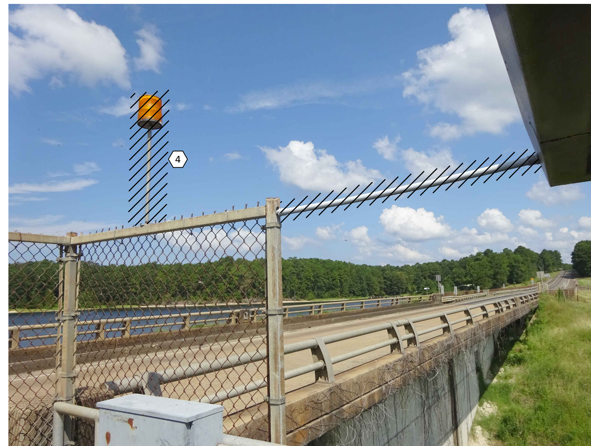
4 GATE 12 BEACON DEMOLITION NOT TO SCALE
