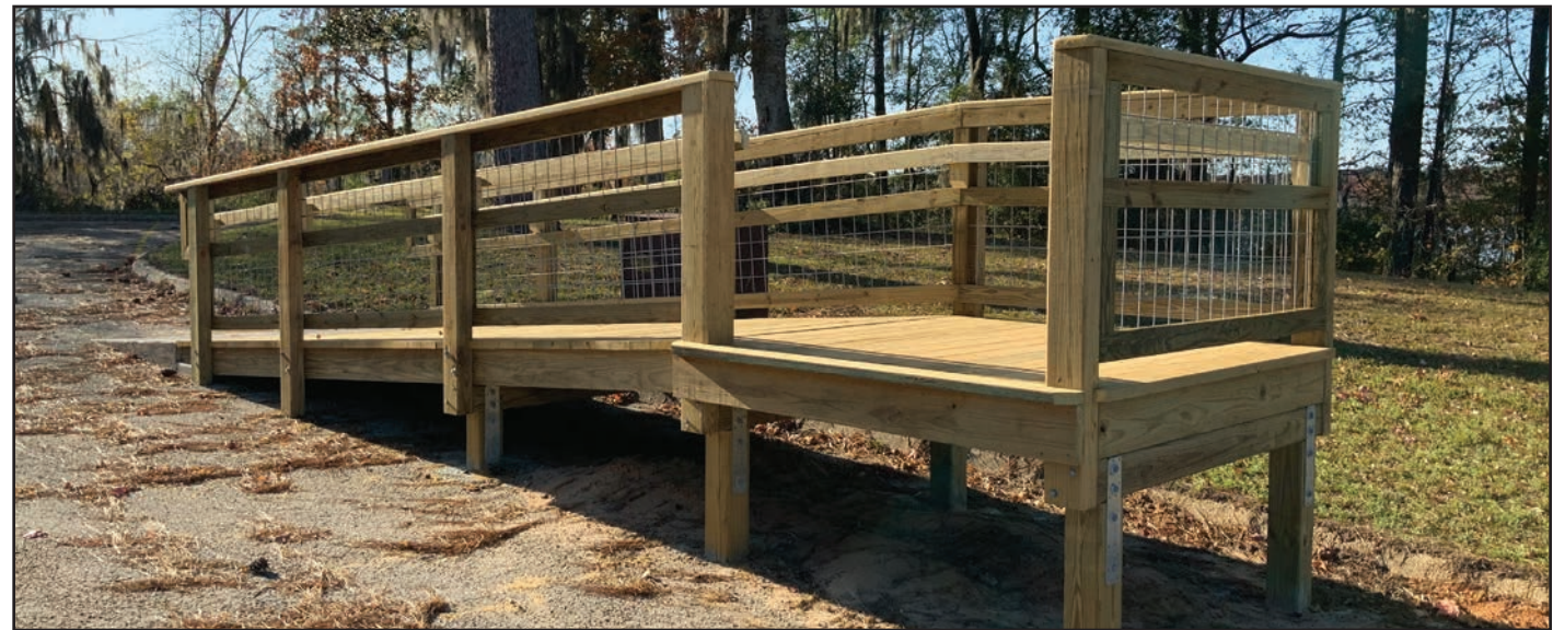
ADA Compliant Wheelchair Ramp for Boating Access at Willow Oak
