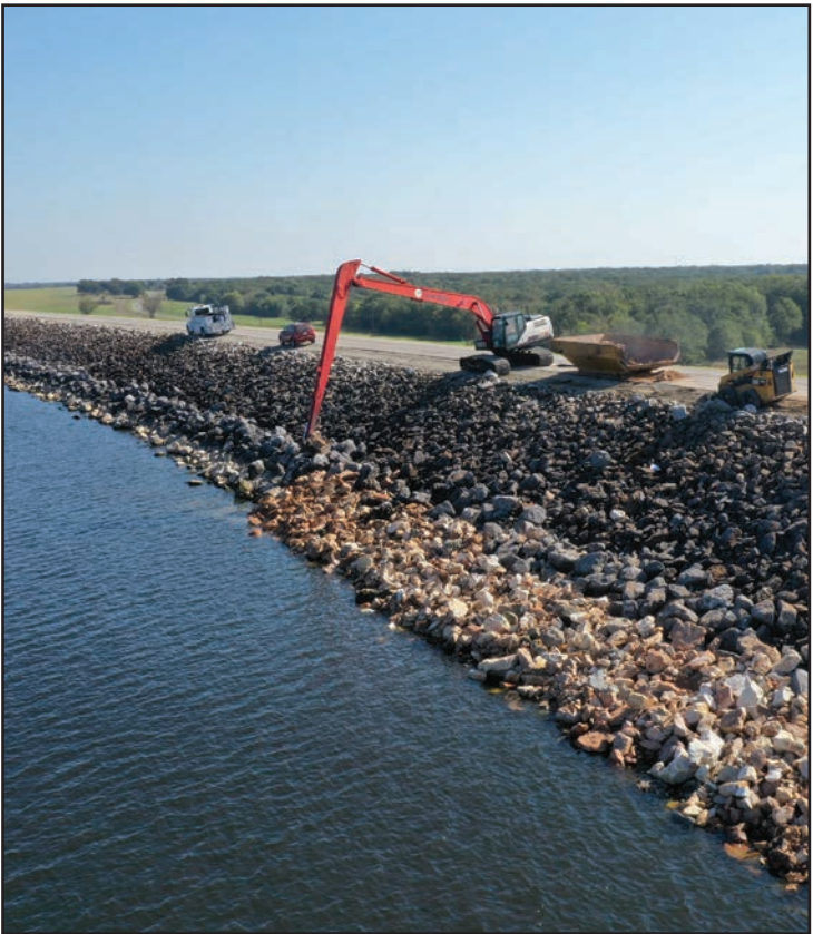
Riprap Replacement on Dam Face
