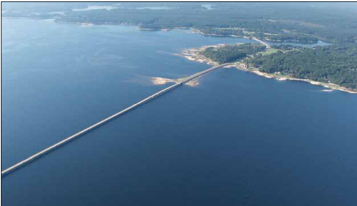
Pendleton Bridge on Toledo Bend Reservoir
