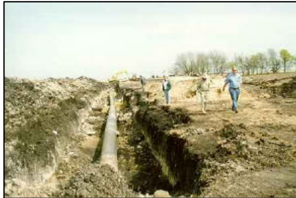
Repaired Section of Ruptured Pipeline
