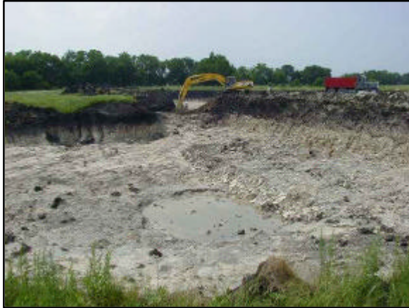
Spill Site Excavation
