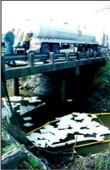
Gasoline Containment and Collection in East Caddo Creek
