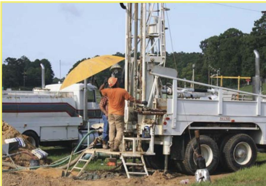
*Drilling New Relief Well Near the Powerhouse*
